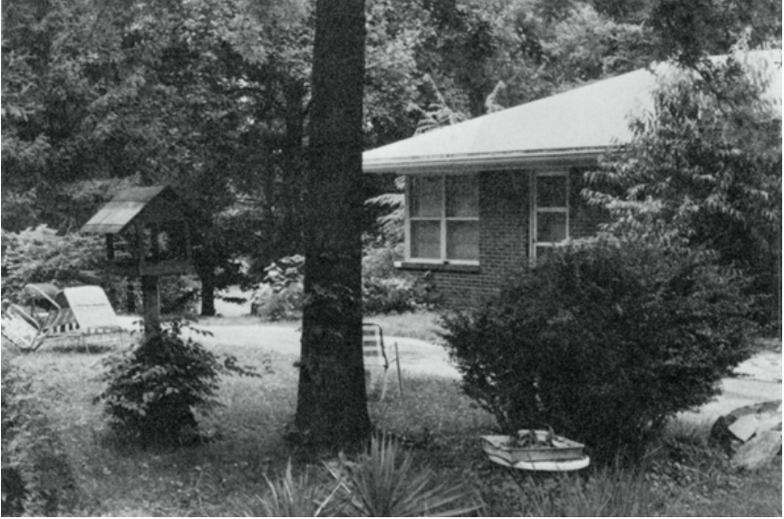
The exterior of the Ra room: the door and corner windows are part of the outside of the room in which the Ra sessions have taken place since January 1981. ( Photo taken June 9, 1982. )
